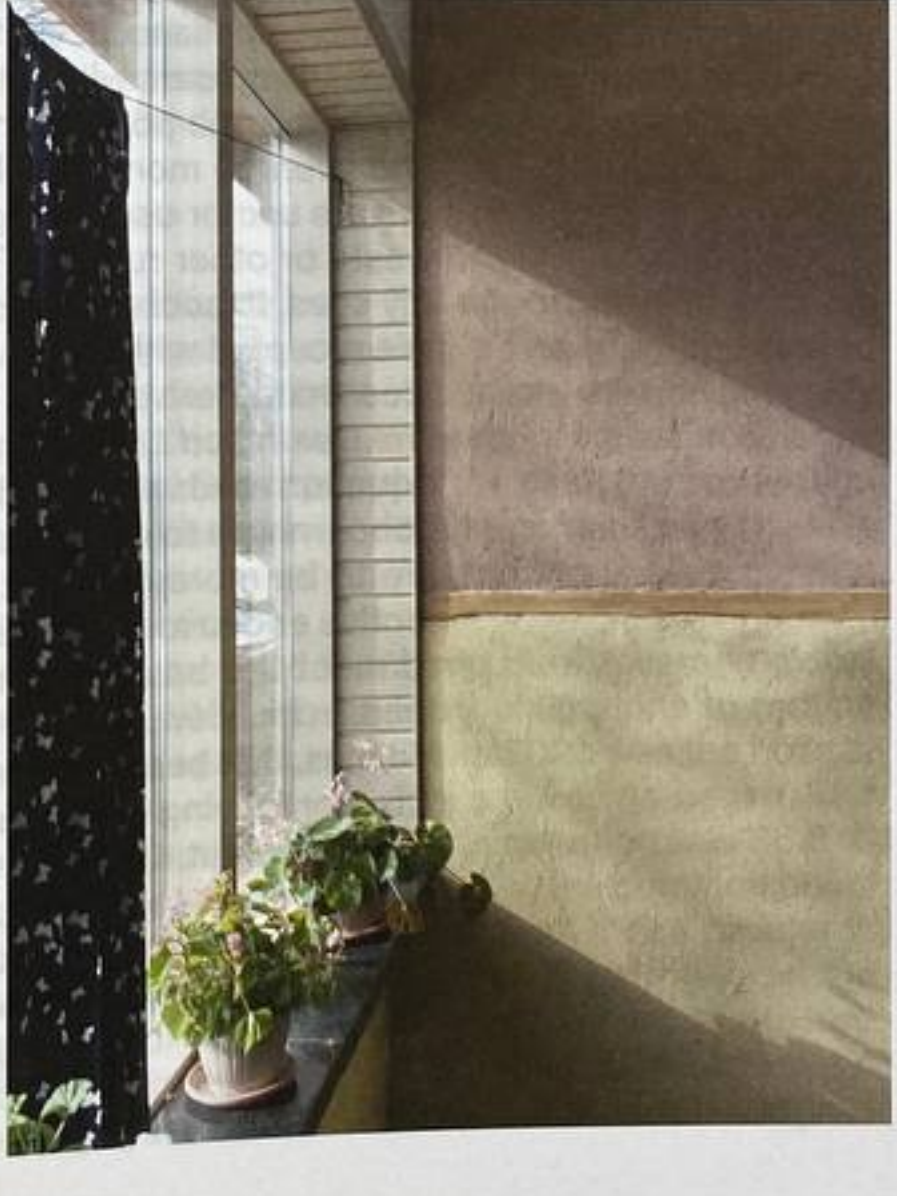
Fig. 5 The interior walls were plastered with 4 cm of coarse clay plaster and then painted with water-soluble paint. The black windowsills covered with plants are of course less effective at receiving and storing the sun's heat.
