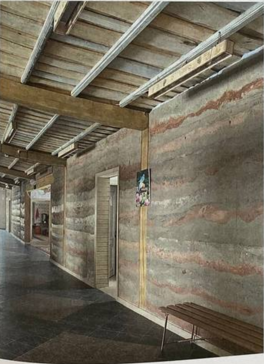
Fig. 4 Rammed-earth wall in the corridor. Inspection one year after completion in December 2023.
