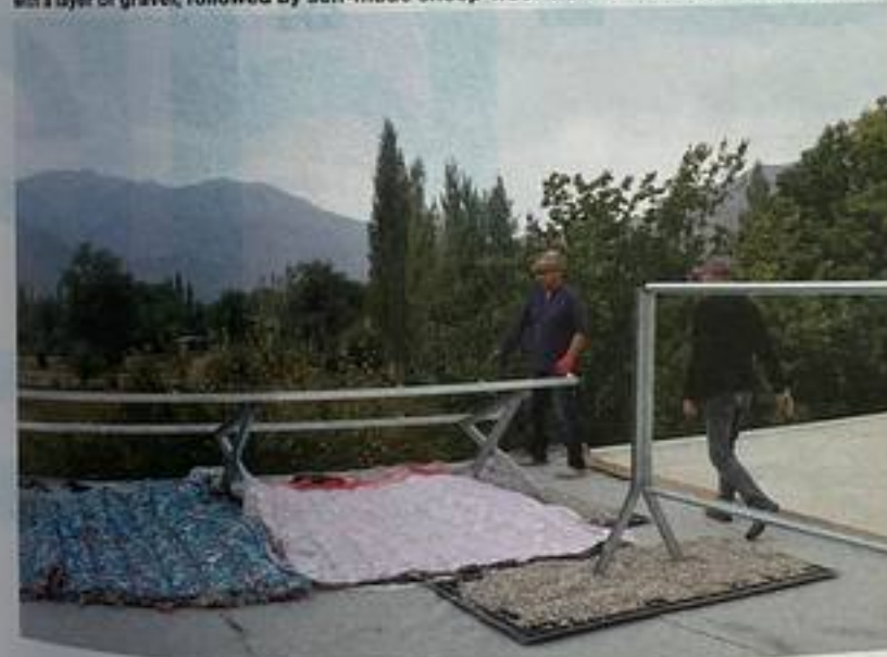
Fig. 11 Installations for the PV system. The base of the construction is stabilised with a layer of gravel, followed by self-made sheep-wool mats as a base for the green roof.
